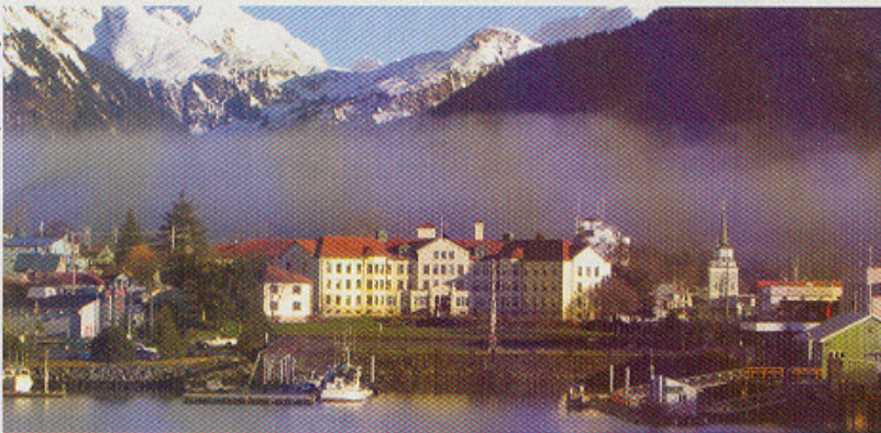
The Sitka Pioneers' Home (large building in center), listed on the National Register, serves as a retirement care center.
